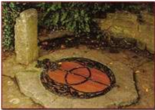
The Well-head is covered by a wooden lid with a fine wrought-iron sculpture.
